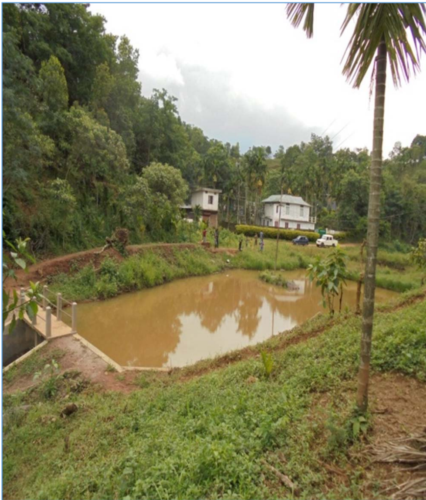
Name of activities :- Water Harvesting structure at Amingokgre. Project: IWMP-XI. Batch – III, Name of watershed: - Balmrik Micro watershed District : West Garo Hills
