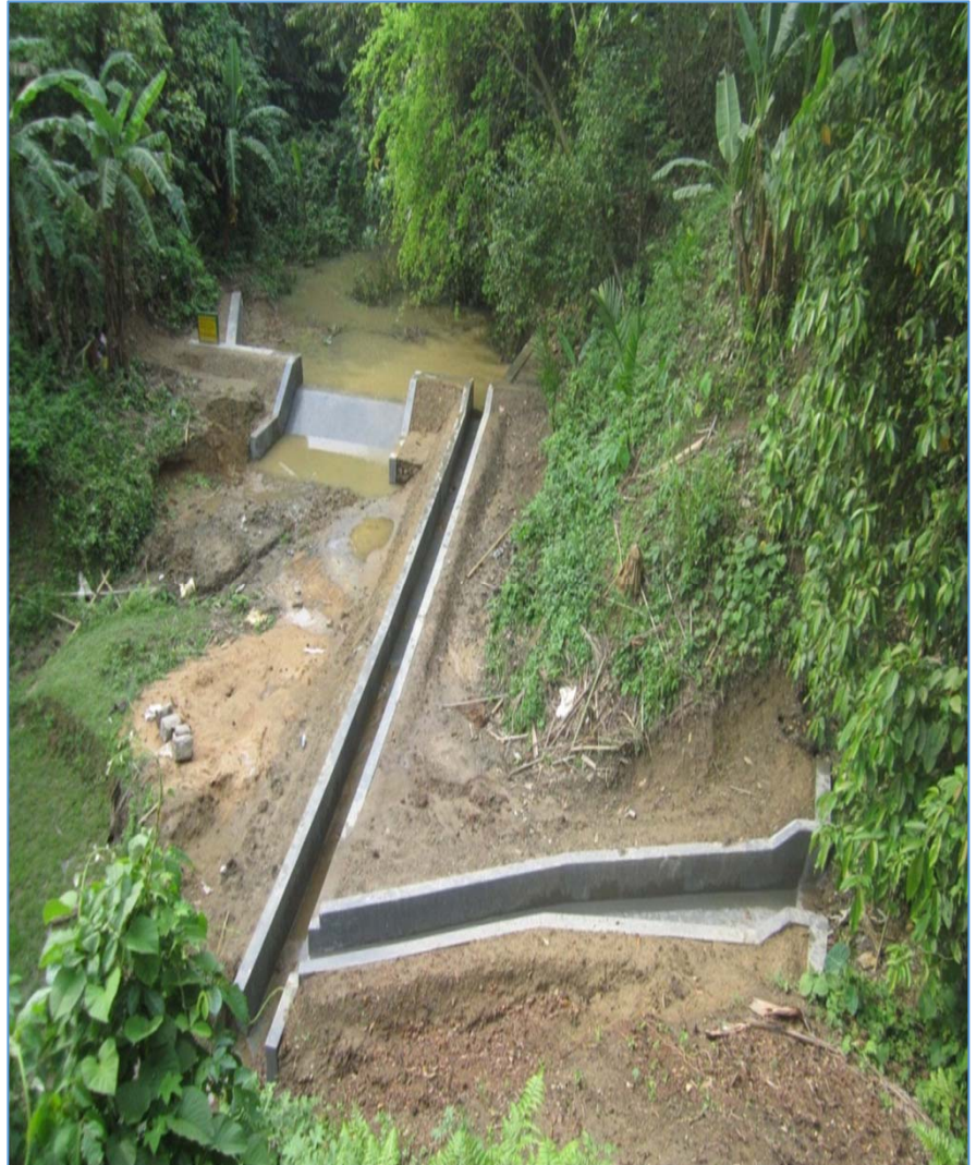
Name of Work: CC Check dam with Channel Name of Watershed : W/shed IWMP Project No XII Batch III IWMP Village : Lower Aju Block : Gambegre C. & RD District: West Garo Hills.
