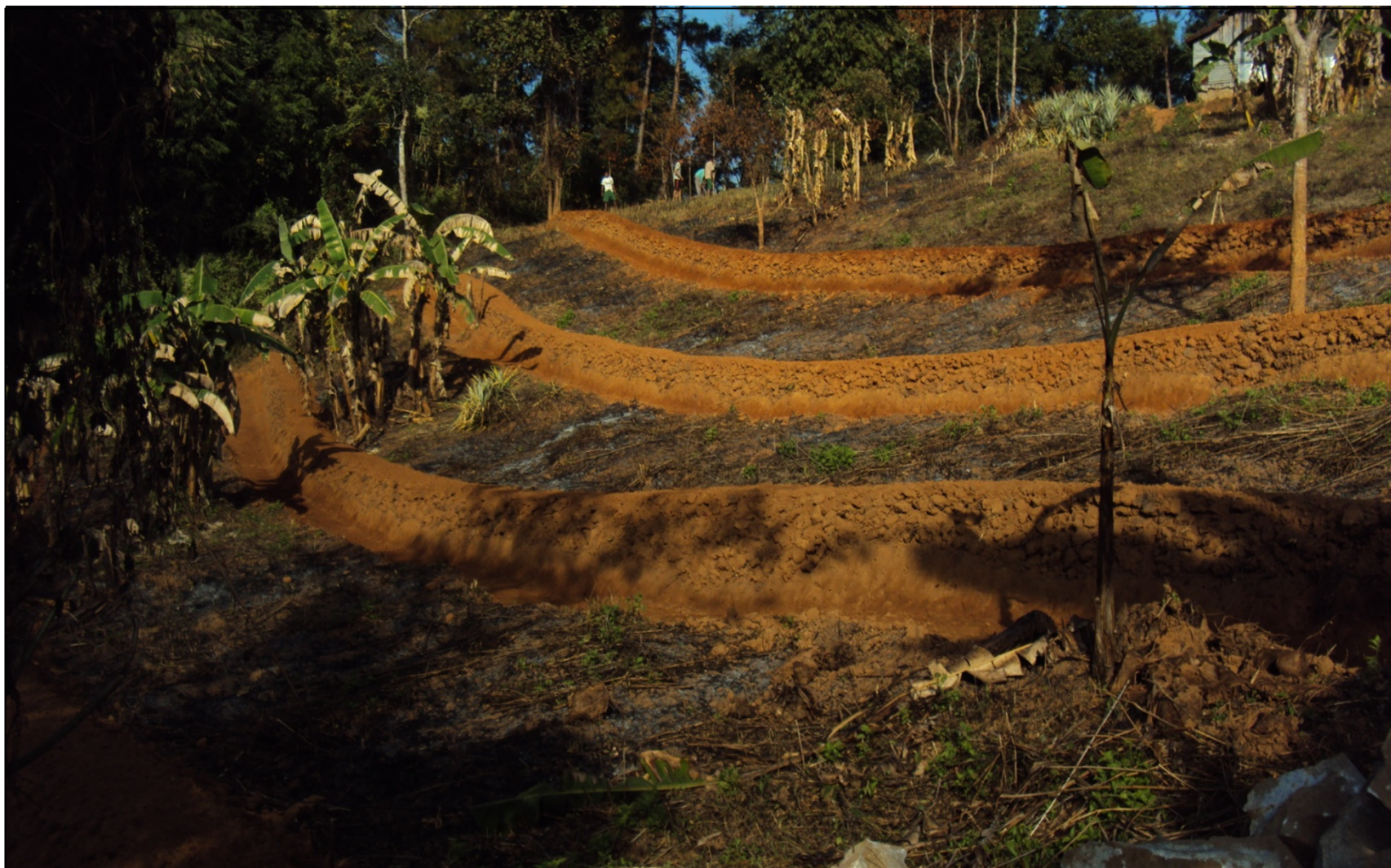
ACTIVITY- COUNTOUR BUNDING,BATCH-II ( IWMP-IV) WATERSHED- LOWER UMPIH WATERSHED VILLAGE- MAWTARI MYRDON C&RD BLOCK-UMSNING DISTRICT- RI BHOI
