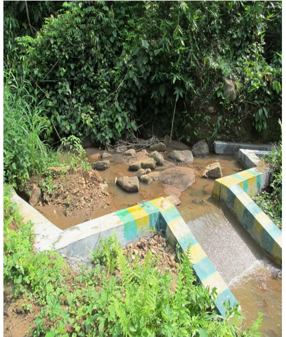
C.C.Dam across Chiko Stream at Samin Indikim under Lower Rongal Watershed, East Garo Hills IWMP-VIII
