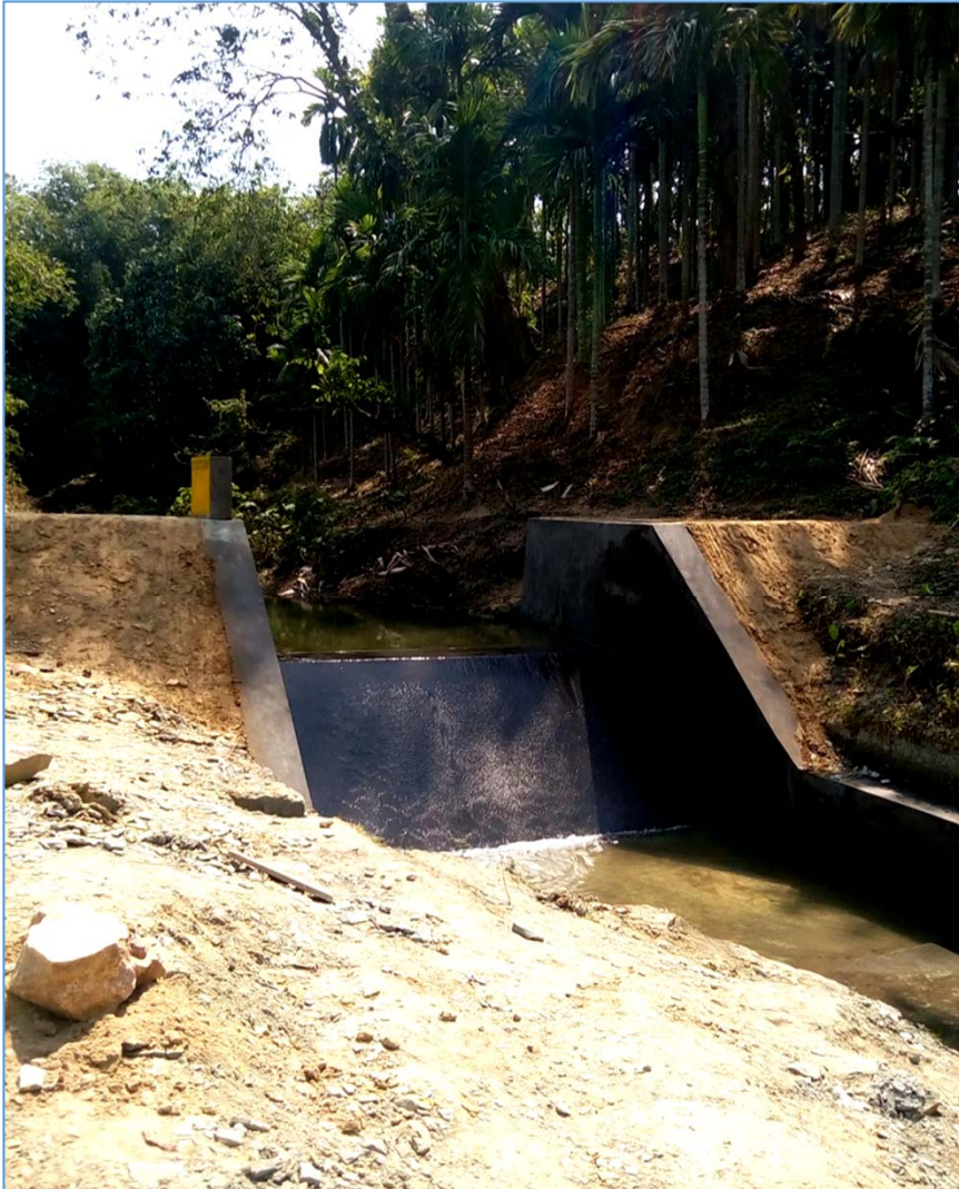
Name of Watershed : Chipra Micro Watershed I.W.M.P. Name of Work : Water Harvesting Structure Project No. XII Batch No. III District : West Garo Hills
