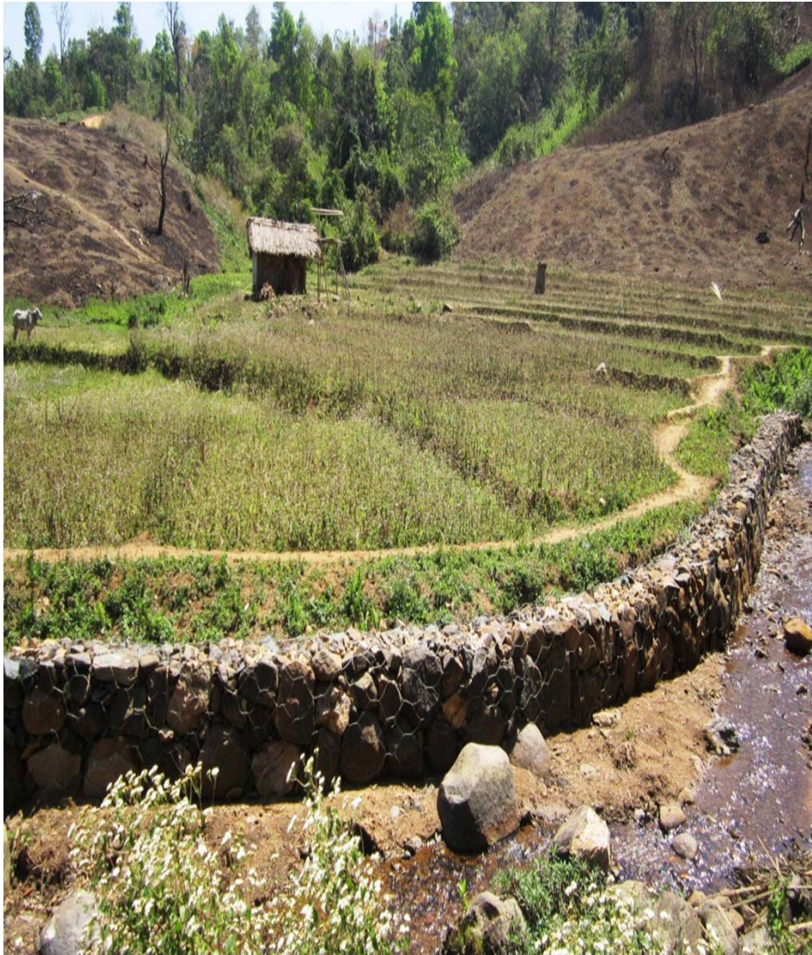
Boulder Sausage Protection wall at Rongal Watershed, East Garo Hills IWMP-II
