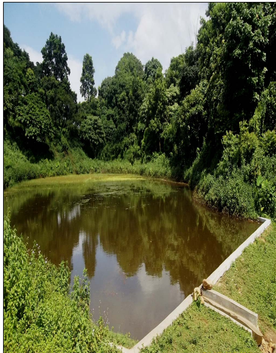
WATER HARVESTING STRUCTURE AT CHIDEKGRE, RINGGI BISIK MICRO WATERSHED , IWMP-V, WEST GARO HILLS
