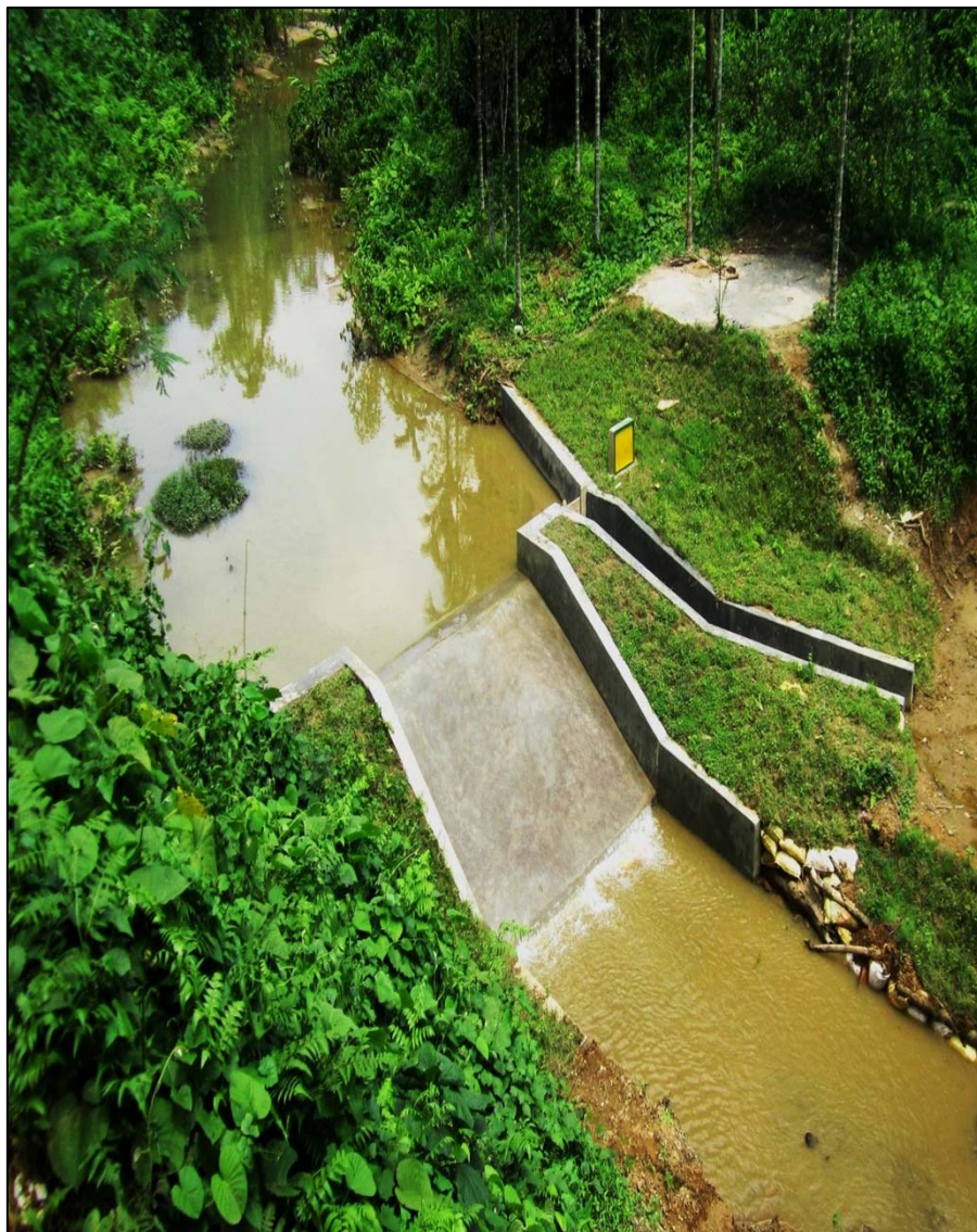
IRRIGATION DAM AT UPPER AJU MICRO WATERSHED IWMP-XII, SANJENGPARA, WEST GARO HILLS
