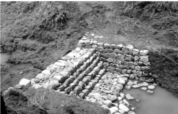
Gully control: strengthening the soil.
