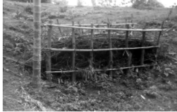
Brushwood check dam
