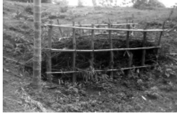
Brushwood check dam
