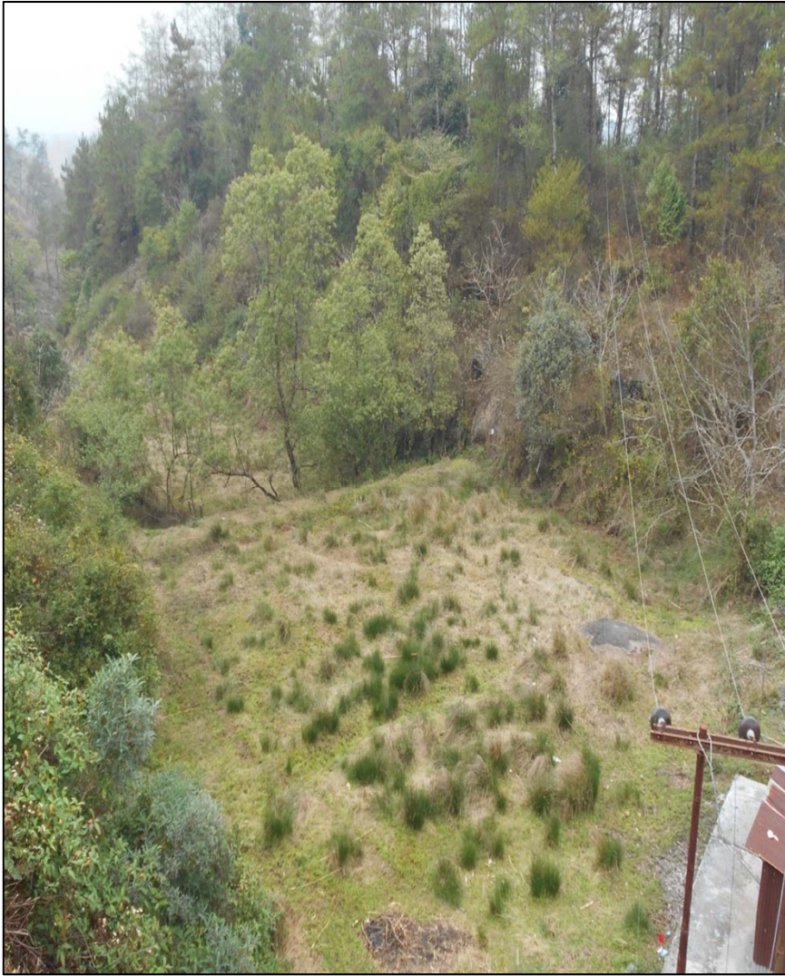
BEFORE CONSTRUCTION AT RANGLANG SOHSYNIANG, SOUTH WEST KHASI HILLS
