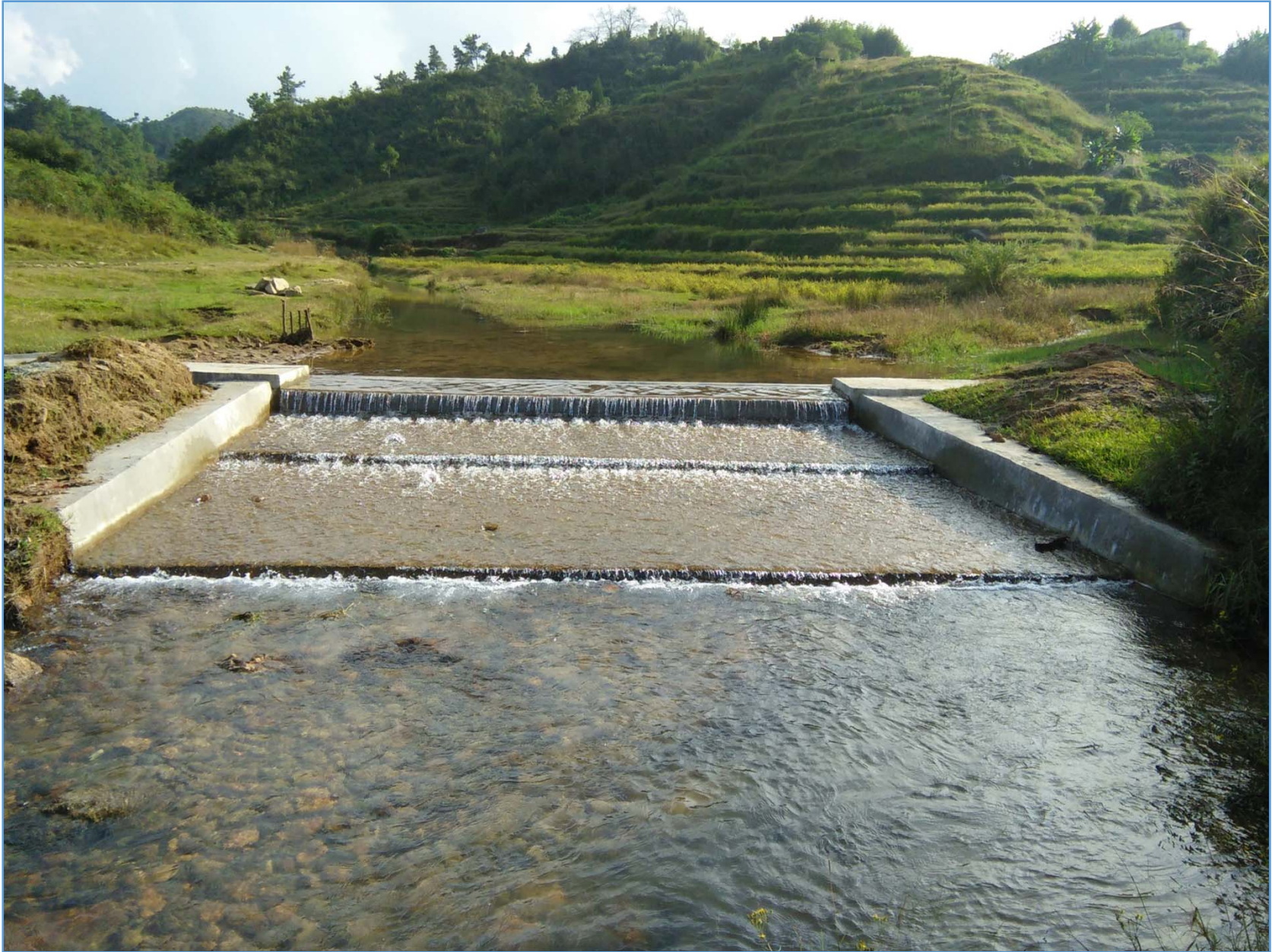
RCC DAM AT UMDIDOH UNDER WAH UMLAWBAH RIDF XX, EAST KHASI HILLS
