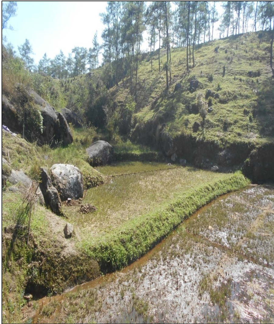
BEFORE CONSTRUCTION AT RANGLANG NONGTYLLA, SOUTH WEST KHASI HILLS
