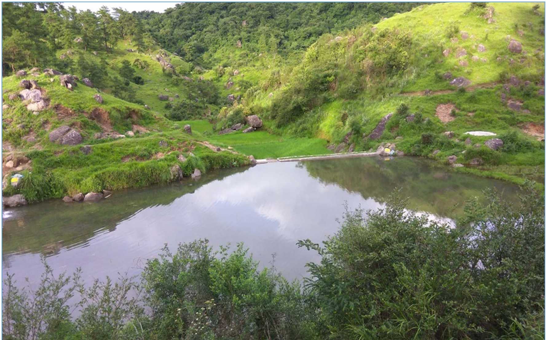
Project: Wahnamlang, RIDF XX Activity: Water Harvesting Structure District: South West Khasi Hills
