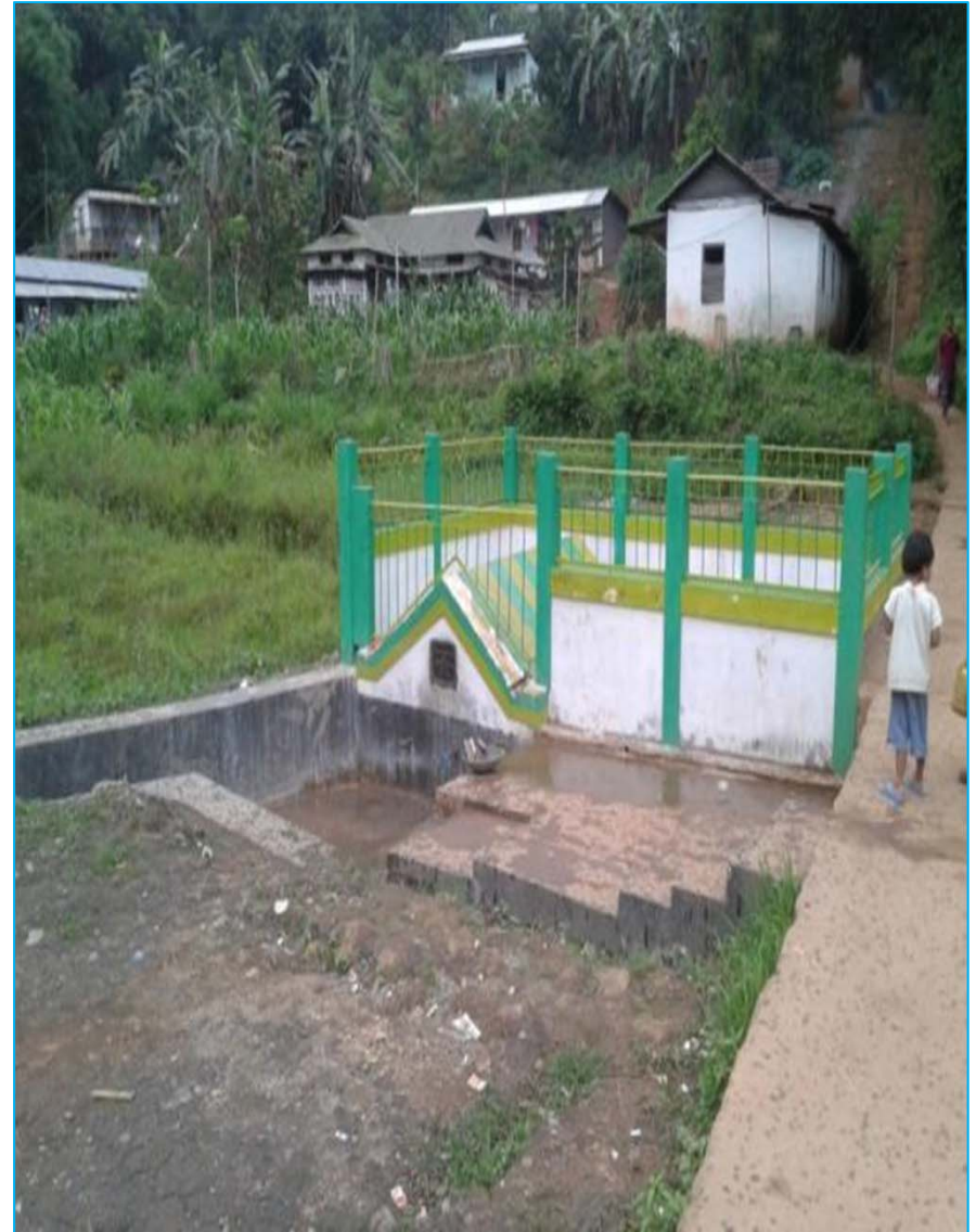
UMHONI-UMPARILA-UMDAIRY RIDF - XX. RCC storage tank for drinking water at Umtarok (Patarim), Ri Bhoi
