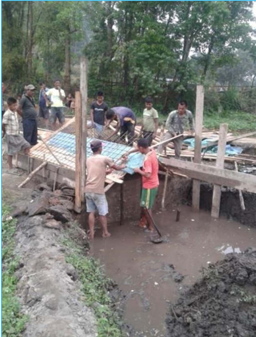
UMHONI-UMPARILA-UMDAIRY RIDF - XX. RCC storage tank for drinking water at Umtarok (Patarim), Ri Bhoi
