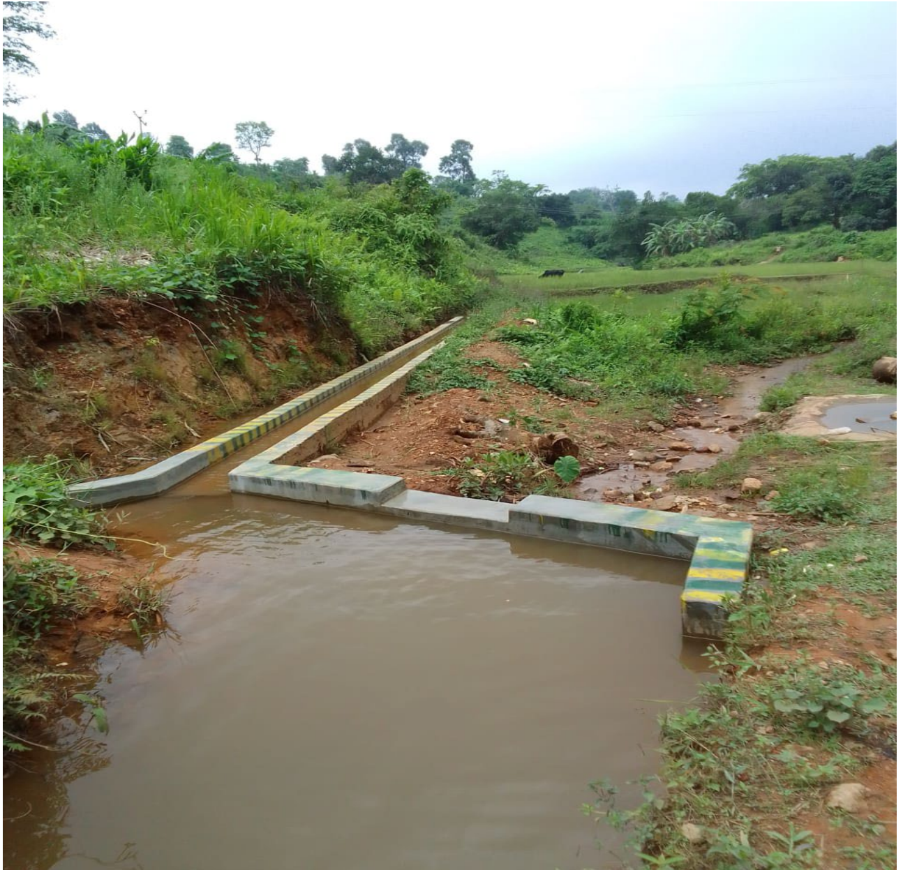
Water harvesting structure at Rongbang
