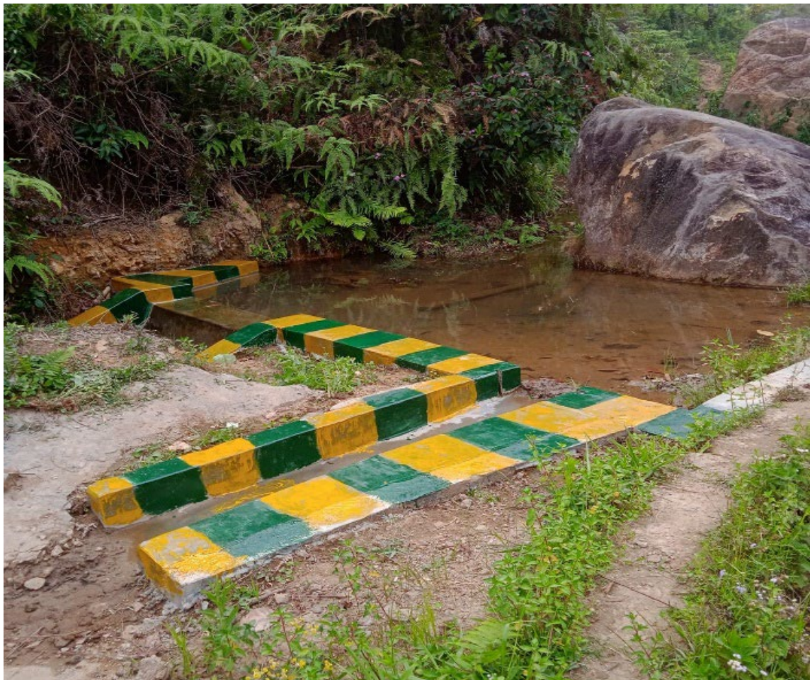
Water Harvesting Structure at Rongbang
