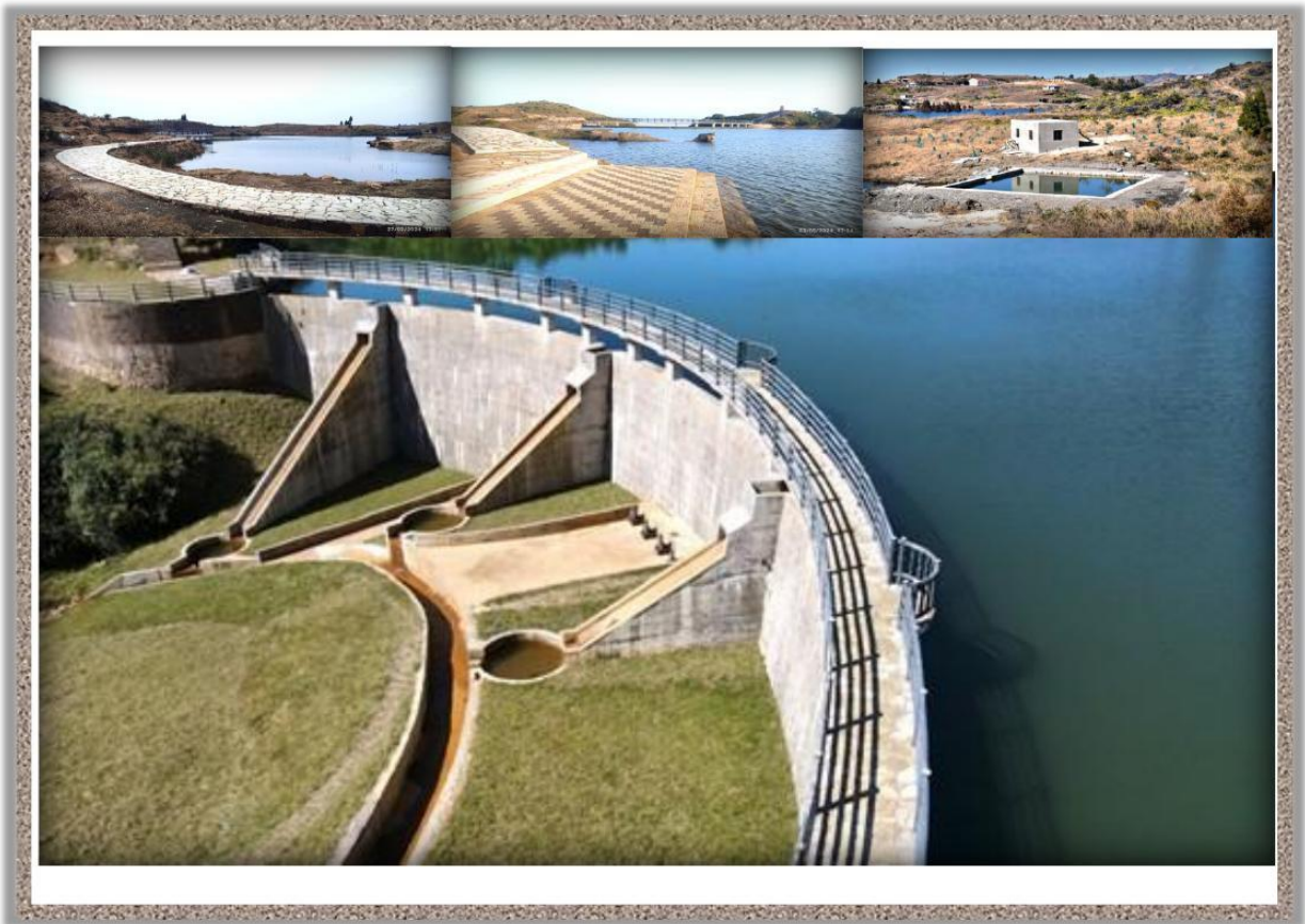
The completed RCC Arch Dam — key civil structure of the reservoir
